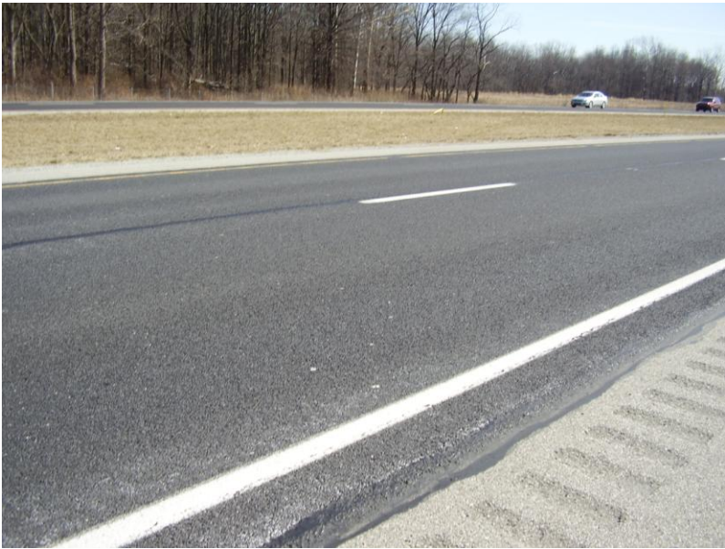
Figure 4.7. Appearance of the PFC Surface after Five Years (3-3-09)
