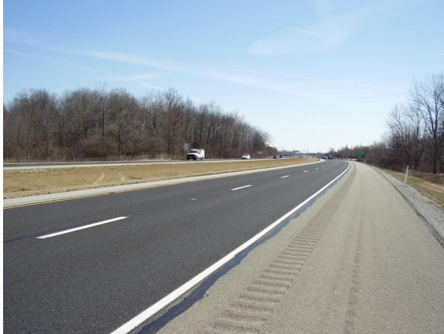
Figure 4.9. Appearance of the SMA Surface after Five Years (3-3-09)
