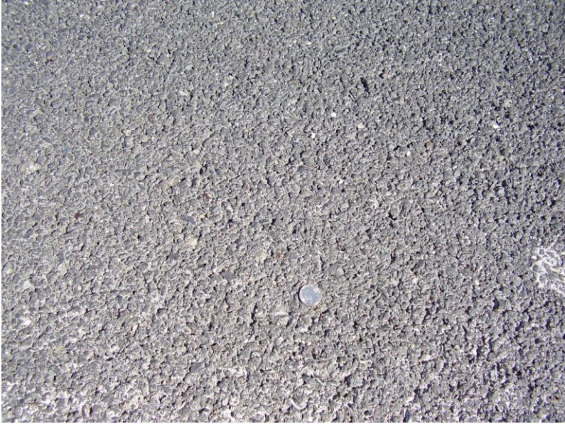
Figure 4.8. Close Up of the PFC Surface Texture (3-3-09)
