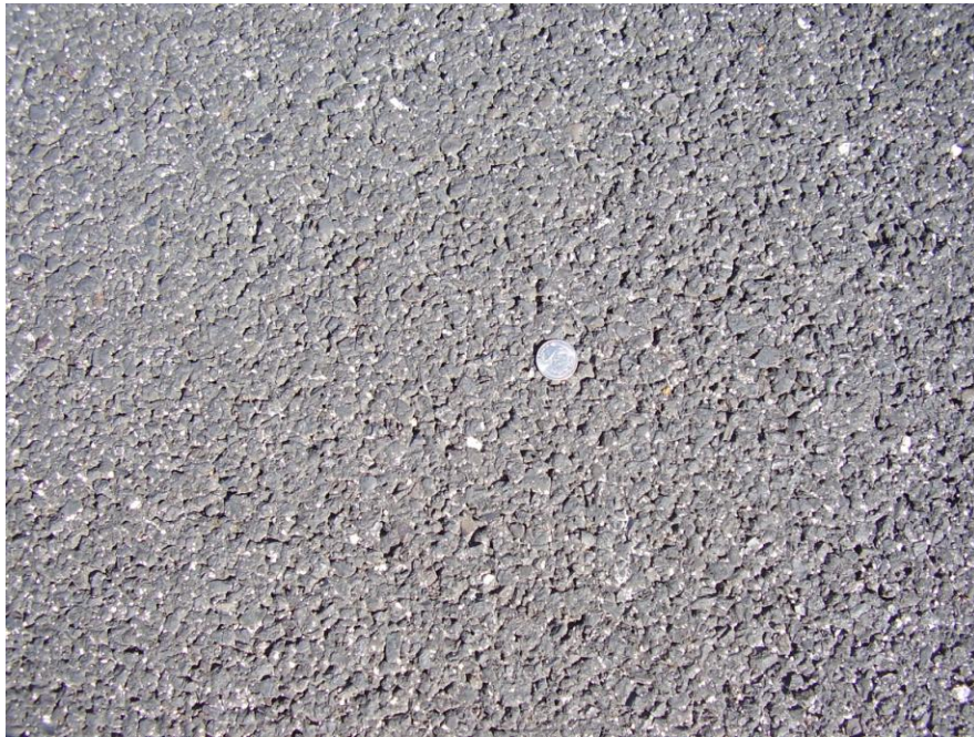
Figure 4.10. Close Up of the SMA Surface Texture (3-3-09)
